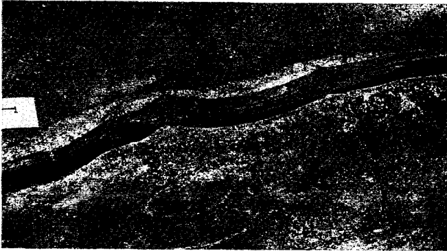
Fig. 6 - Open Crack at stiffener ring
